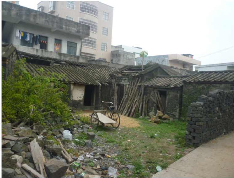
Figure 1 – Old and New Housing in Rural Haikou, Hainan Island, China (Source: Ali Cheshmehzangi, February 2014)
